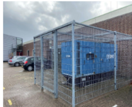
Emergency power generator
