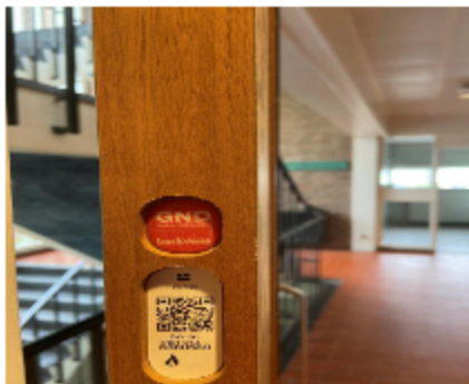
fire rated door
