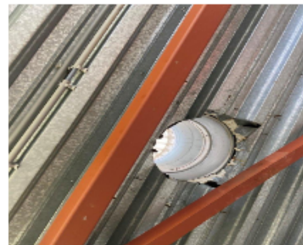
roof penetration (RI)
