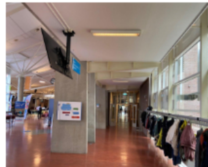
Concrete/ steel construction
