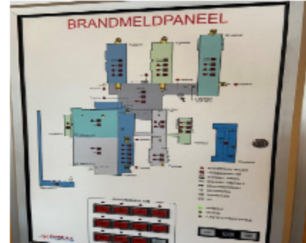
Fire alarm panel
